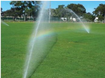
Sprinklers and filtration system being tested during commissioning and hand over of the newly installed irrigation system.
