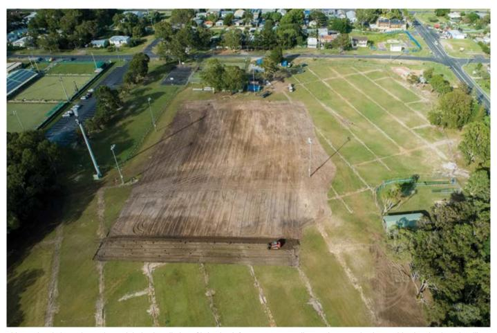
This overhead photo shows the oval during installation of irrigation infrastructure, as well as oval surrounds. The machine is using laser levelling to cut and fill the surface of the oval. The pipes and risers are already installed.
